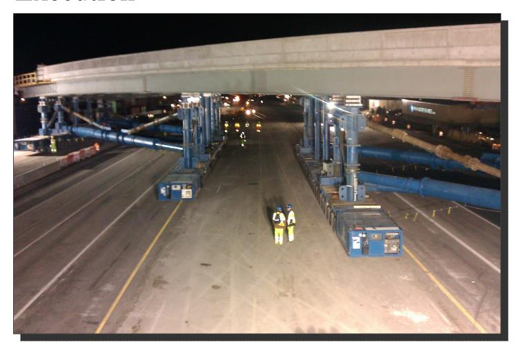
**ONE-NIGHT TRANSPORT** Freeway is closed, barrier is removed, and transitions are constructed. Bridge is then transported, rotated, and set down in a mere few hours.
