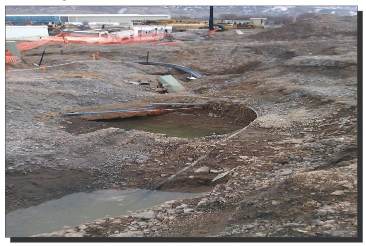
Depending on type, depth, and location of the utilities, additional plates, fills, and route adjustments are established to protect the third party utilities.
