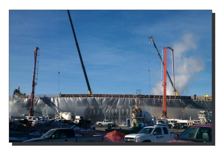
Due to the bridge being built offline, the deck can be fully tented, heated and easily accessible even in the winter. Because of the access, the deck was also poured with two Bidwell machines reducing the pour duration in half.
