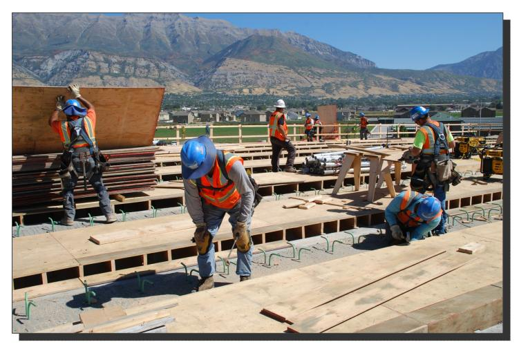
DECK POUR AND SCREEDS As the bridge is built in a different location with differing elevations, the screed elevations are modified to match the called-out screeds once the bridge is placed.
