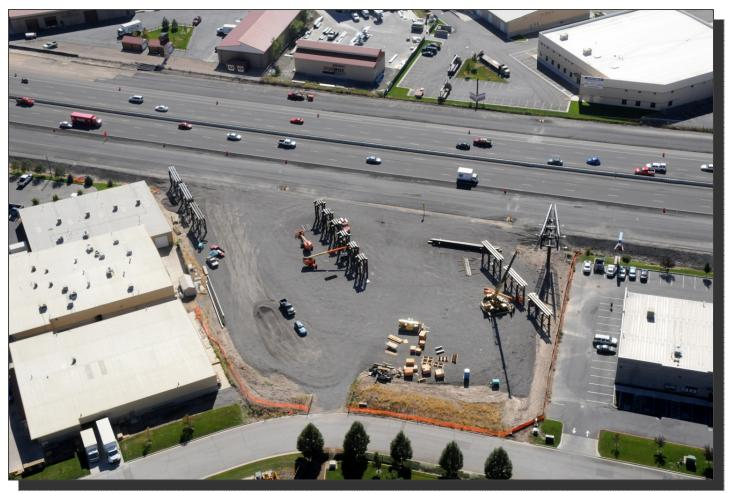
H-pile temporary abutments driven over 90 feet then constructed of 14 x 89 H-piles with cross frames and headers for beam seats.
