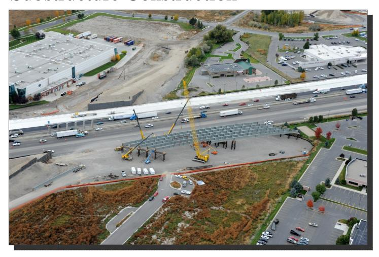
Pile caps, abutments, and columns are constructed in the same manner as conventional.
