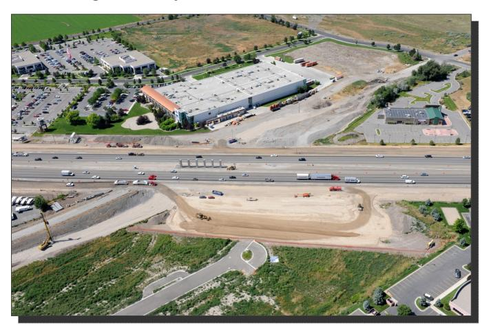
Design delta is established; the initial grading and alignment is determined for construction of the temporary abutments. Geotechnical engineer evaluates soils and ground pressure to determine material requirements for bridge farm.
